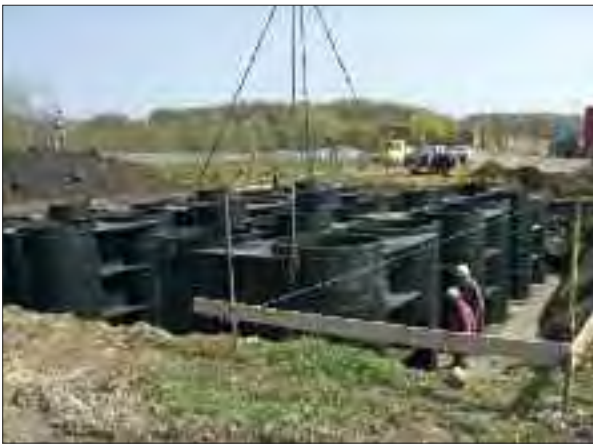
Lysimeter station under construction
