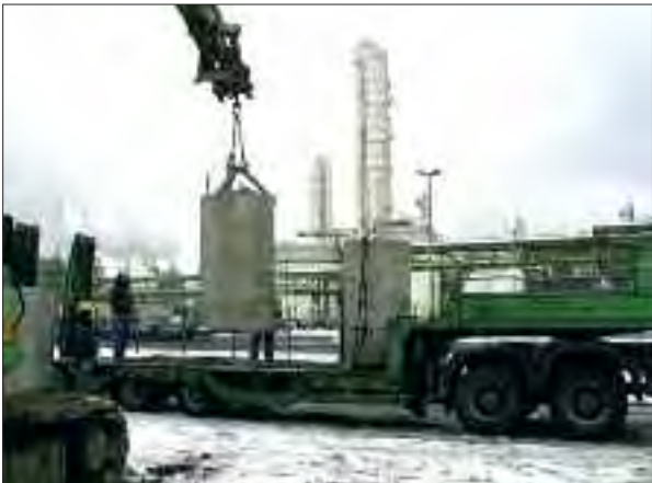
Loading and transport of the cut soil monoliths
