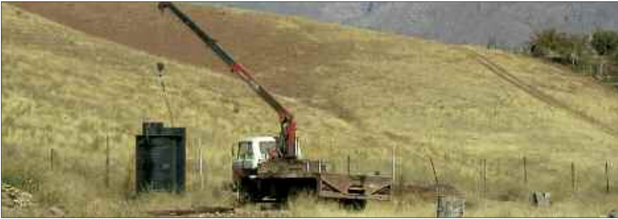
Installation of the PE-HD lysimeter station
