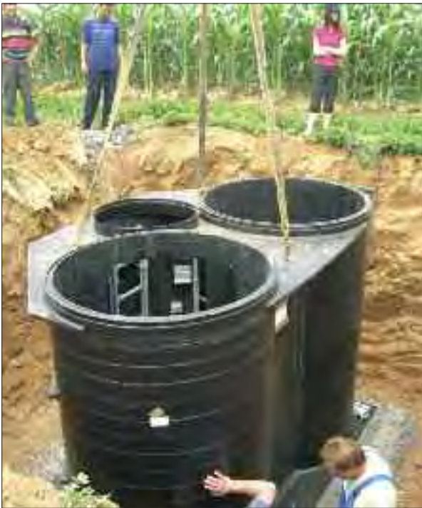
Installation of the 2-fold lysimeter station
