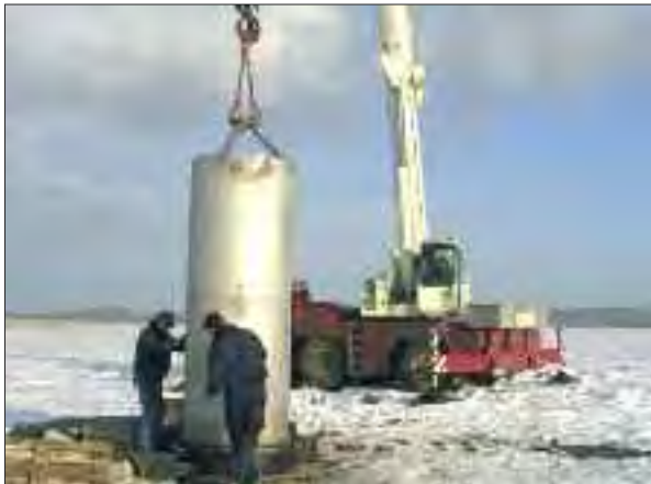
Insertion of the lysimeter in the station
