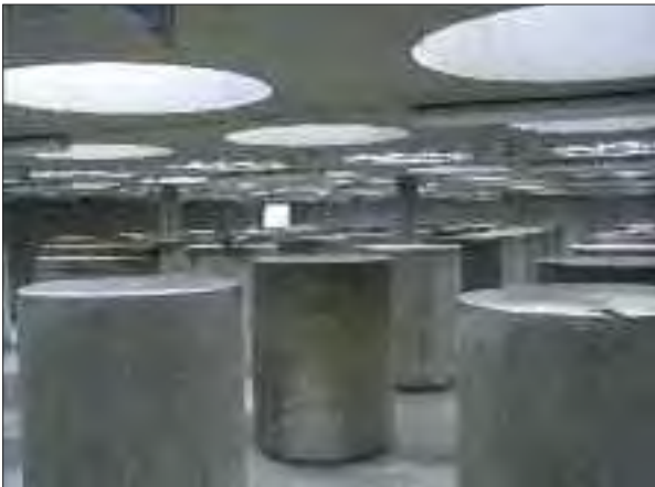
Costruction of the basement for the lysimeter station
