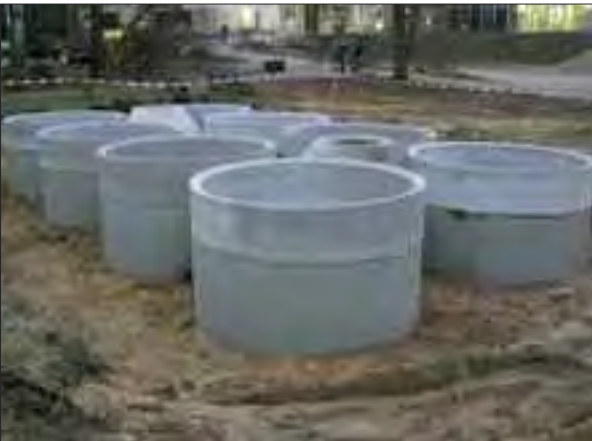
None containerized concrete lysimeters under construction
