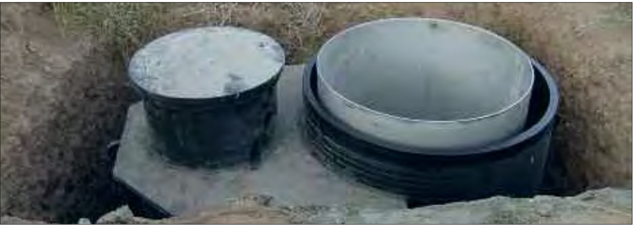
Containerized Lysimeter station during the installation works
